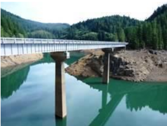
Whatcomb Bridge Preservation
